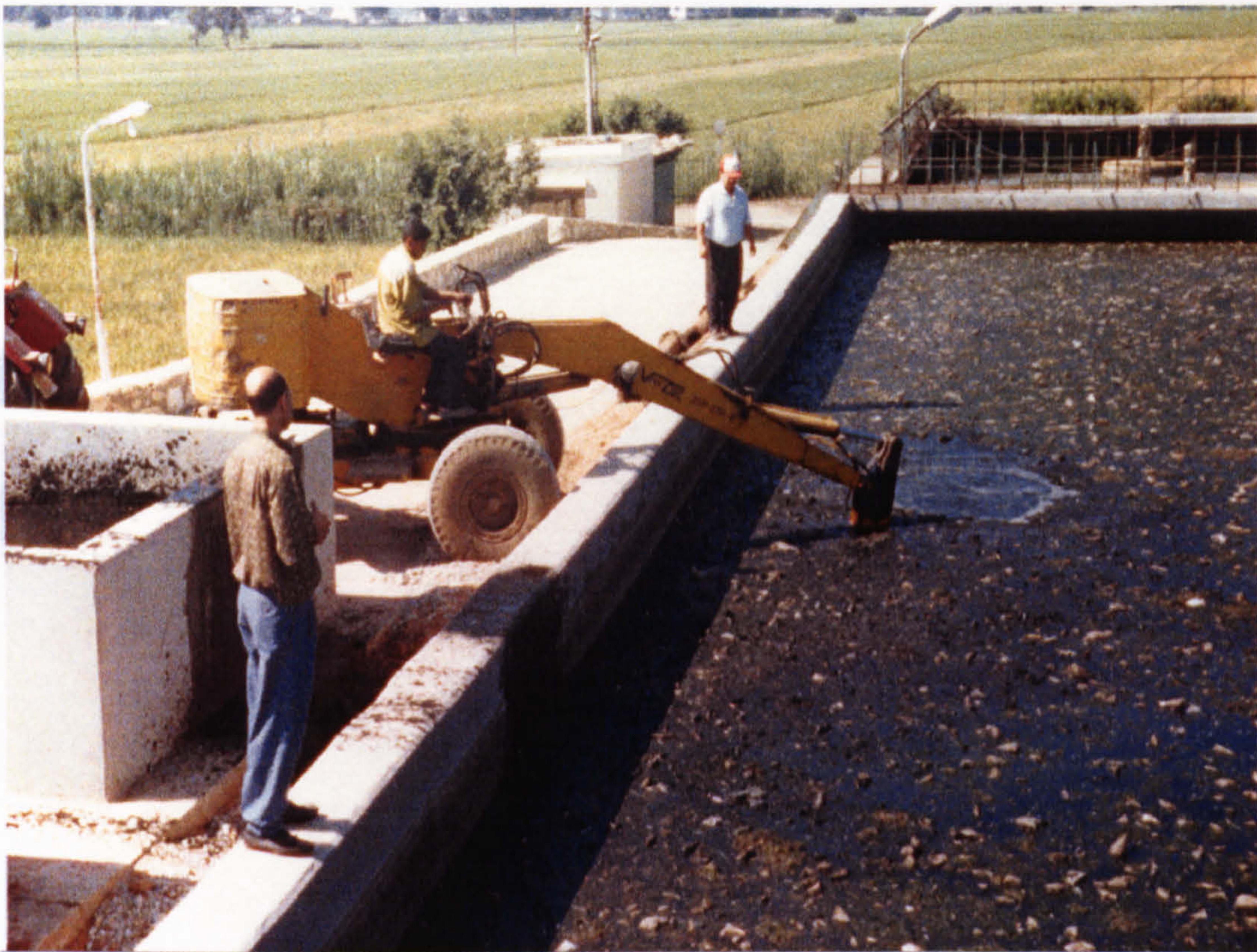
Figure 3.4. Anaerobic Pond Sludge Transported to Drying Beds using an Excavator
