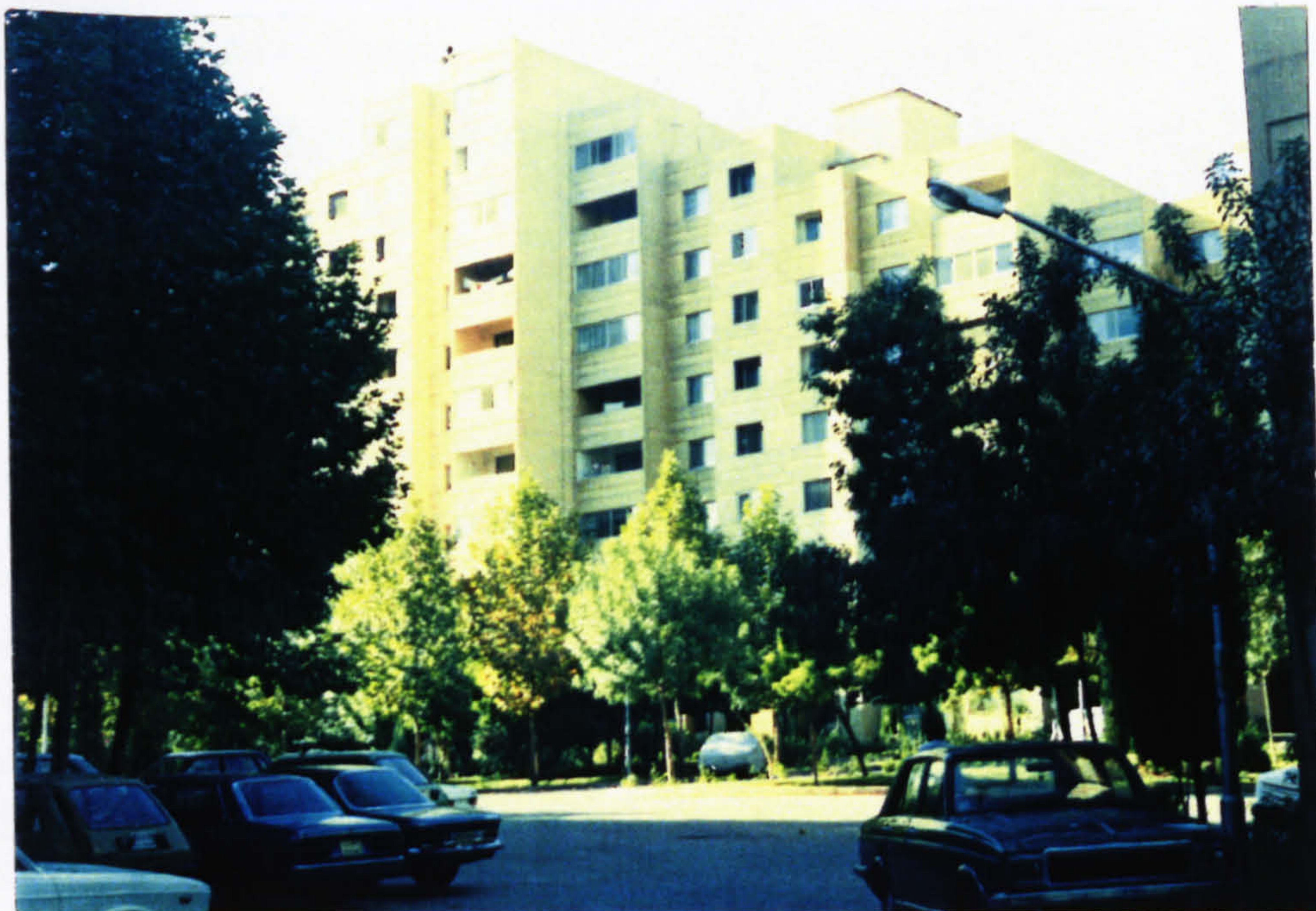
Figure 6.2 The external structure of housing in Apadana
