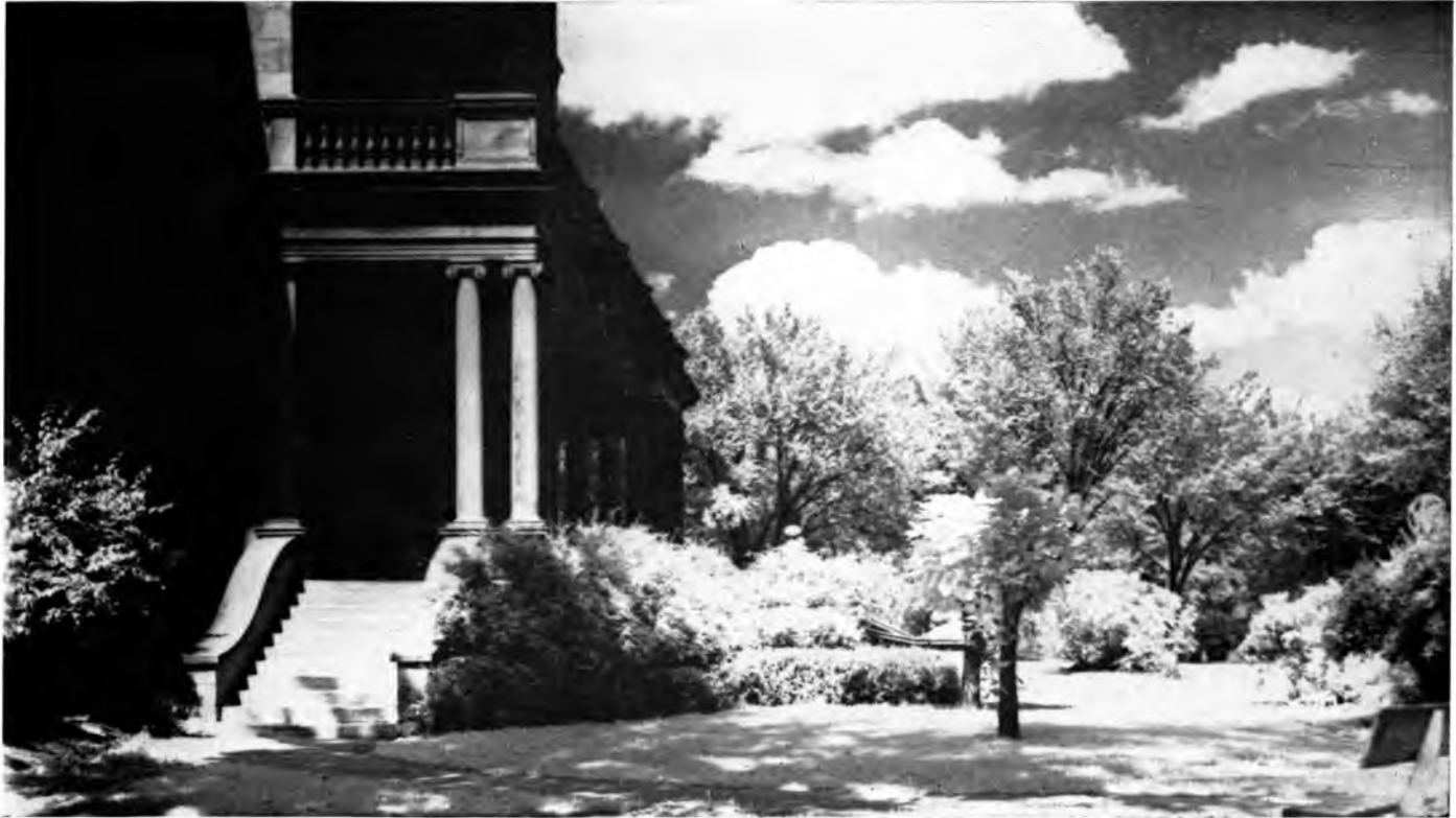
ADMINISTRATION BUILDING PORTICO
