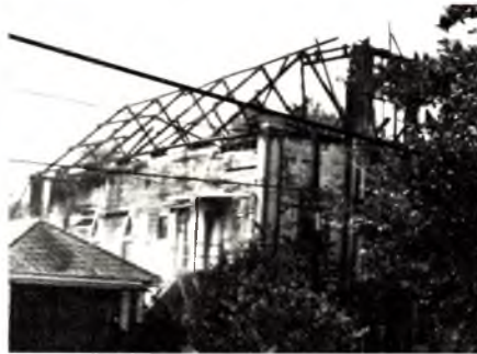
The gutted frame building that served as home for New Orleans Filadelfia church.
