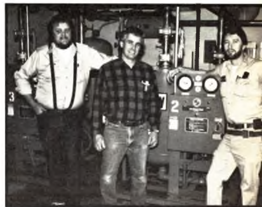
Denny (center) is joined by two of the men he worked with while installing a vacuum system at Kansas City's Children's Mercy Hospital.
