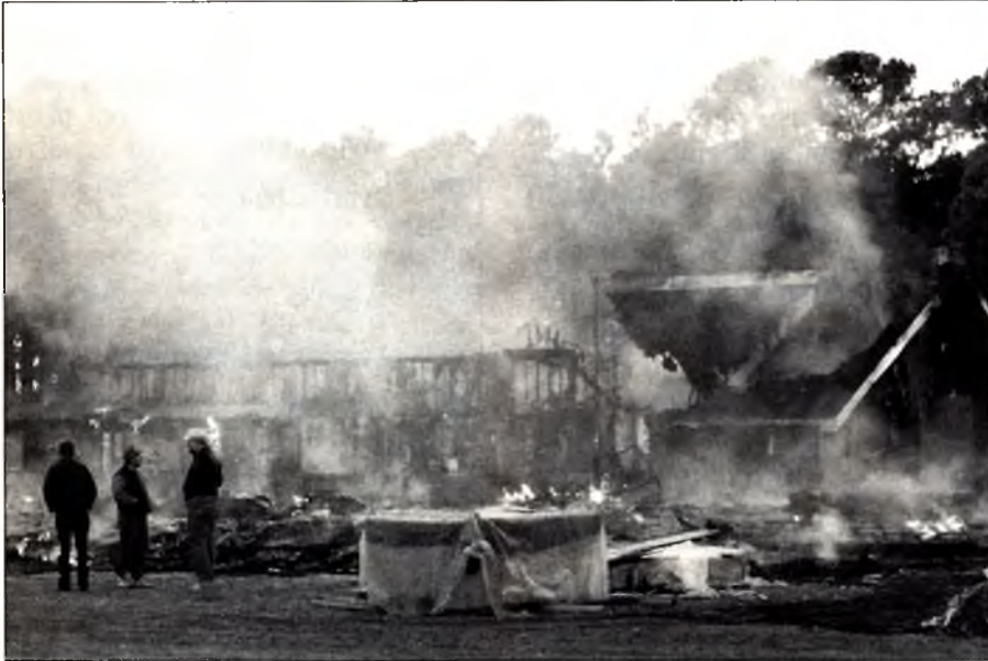
The shell of what once was the building for the Crystal Coast Church of the Nazarene in Morehead City, N.C.
