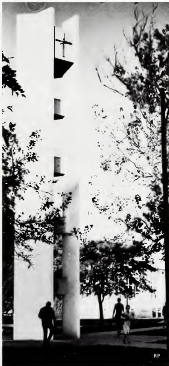
A restoration process has begun this year on Milby Clock Tower.
