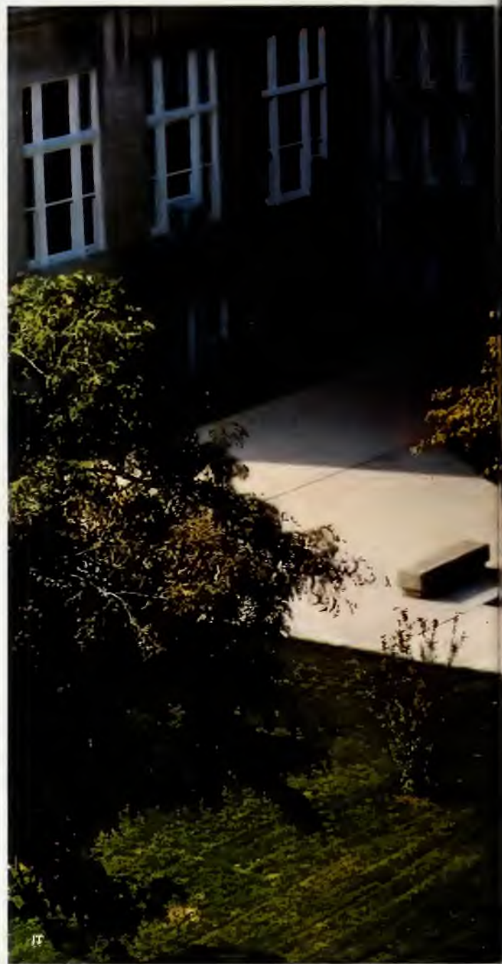
The academic center of the campus, Burke Administration Building, bustles with activity during the day.
