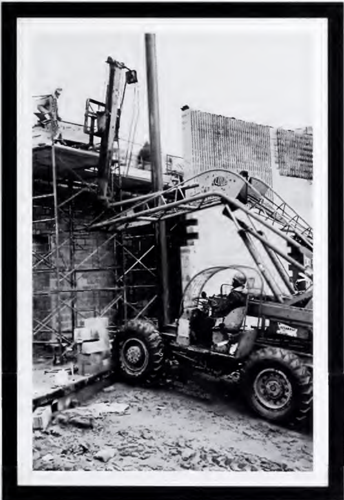
Azzarelli Construction Sites On Olivet's Campus
