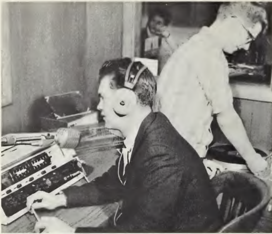
Supervisor Rich Ungerbuehler monitors the controls.
