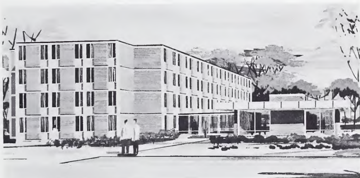
Willingham Hall (under construction)
