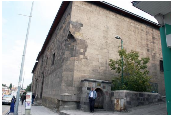
Figure 4.The west side of Ulucami (Original, 2006)
