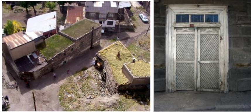
Figure 10. A sample of earthen roof (Original, 2006) and a sample of tırhiç (Original, 2006)
