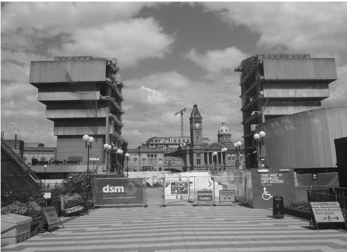
13. Demolition of central library, 2016
