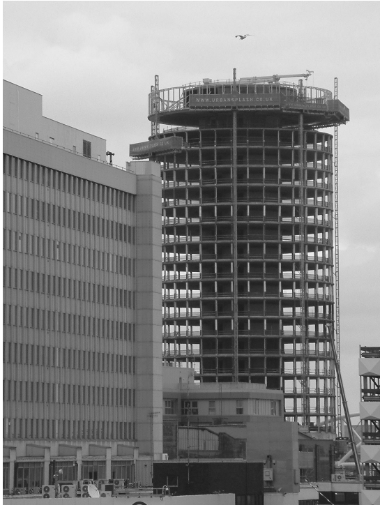
20. The Rotunda, stripped for refurbishment, 2006 (more standard reconstruction-period building to left)
