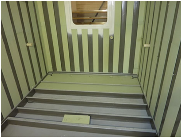
Fig. 6. The steelwork of each container was constructed first. Photo: JM Services
