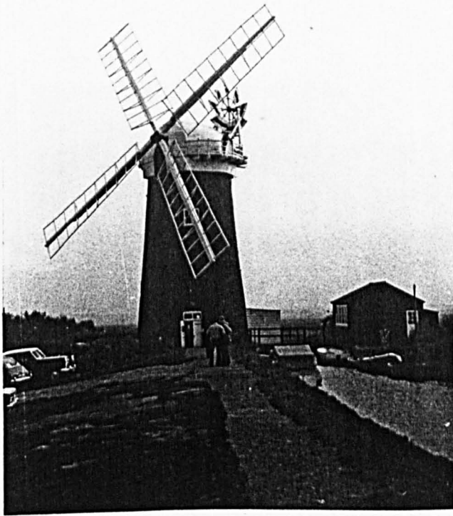
Fig 5.6: North European traditional windmill (English type) showing lattice framework over which 'Common sails' are stretched when working.
