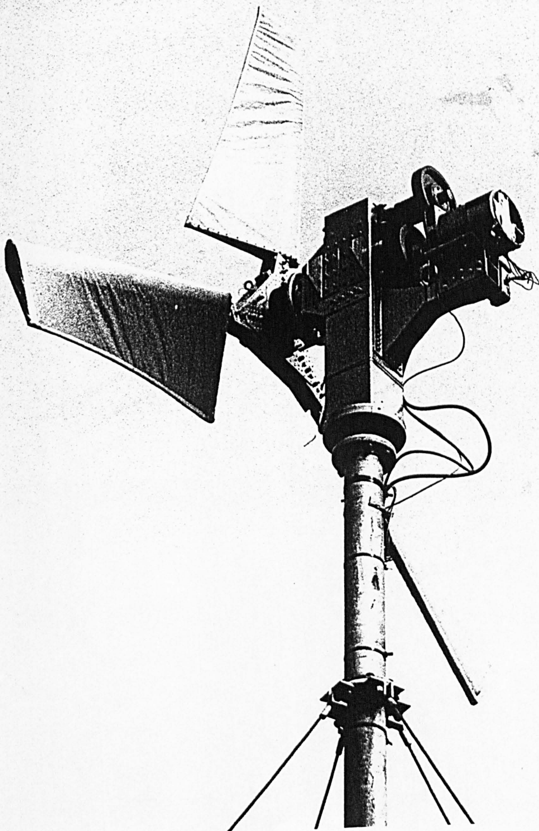
Figure 8.1: View of wind turbine at head of mast showing transmission arrangement with generator on chassis able to rotate about vertical axis (yaw)
