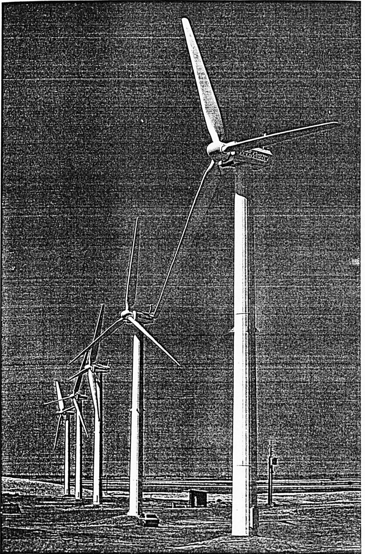
Figure 3.20: Wind farm in California
