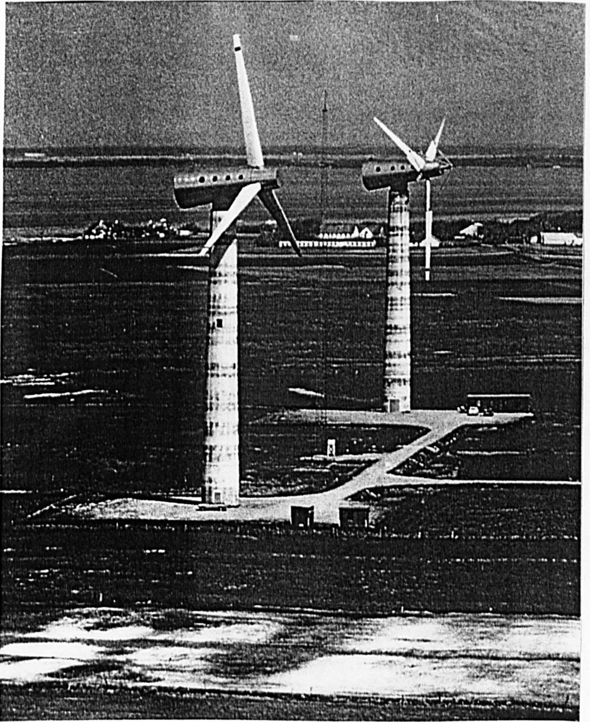
Fig 3.19: Two 40 m diameter 630kW HAWT generators at Nibe, Denmark
