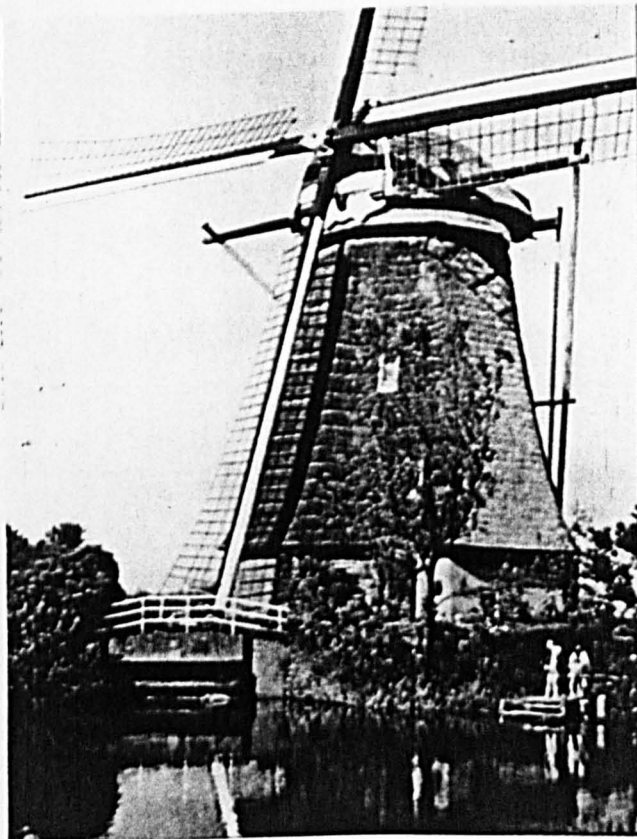
Fig 5.7: Traditional windmill (Dutch type) showing slightly different lattice framework for sails.
