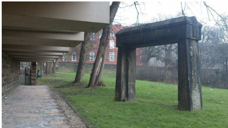
FIGURE 5. Filled-in Arch in St George's Field 2014. This arch forms part of the cemetery wall and faces onto Clarendon Road and an area known as Woodhouse Moor. There is also a campus vehicle exit road nearby, Cemetery Road. The building on the left is the Henry Price halls of residence. © Tina Richardson
