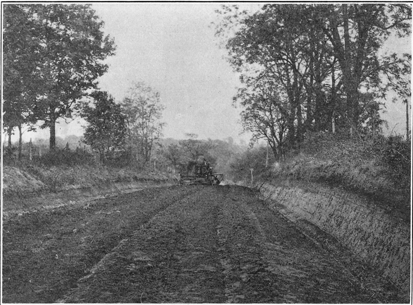
FIG. 30.— Final Round of Grader.
