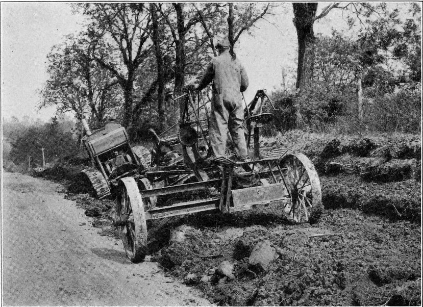
FIG. 22.— Third Round With Grader.
