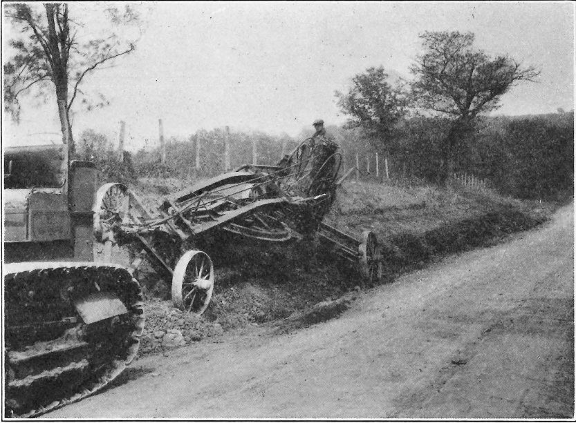
FIG. 31.—Cutting Down High Bank.
