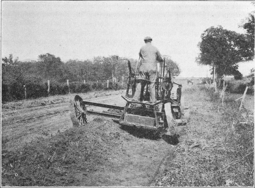
FIG. 4.— First Cut With Grader.
