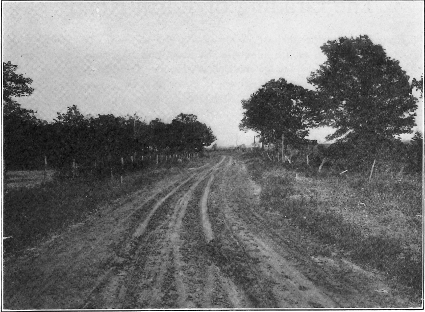
FIG. 2.—Road immediately before grading.
