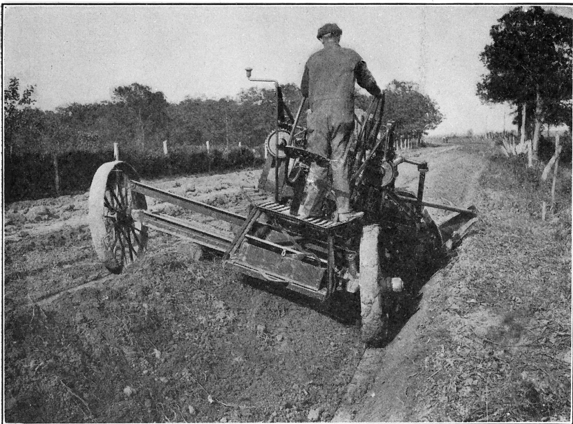
FIG. 12.— Seventh Round of Grader With Back-Sloper Attached. Rear View.
