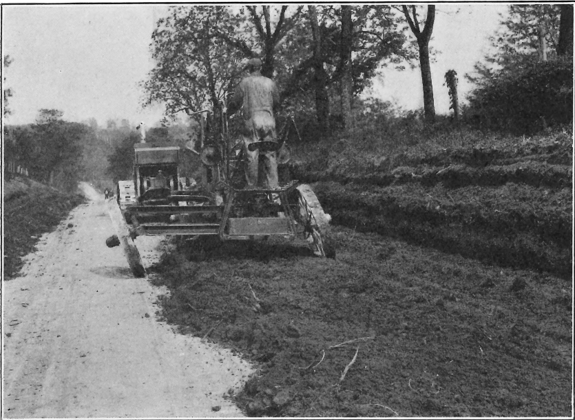
FIG. 24.— Fifth Round With Grader.
