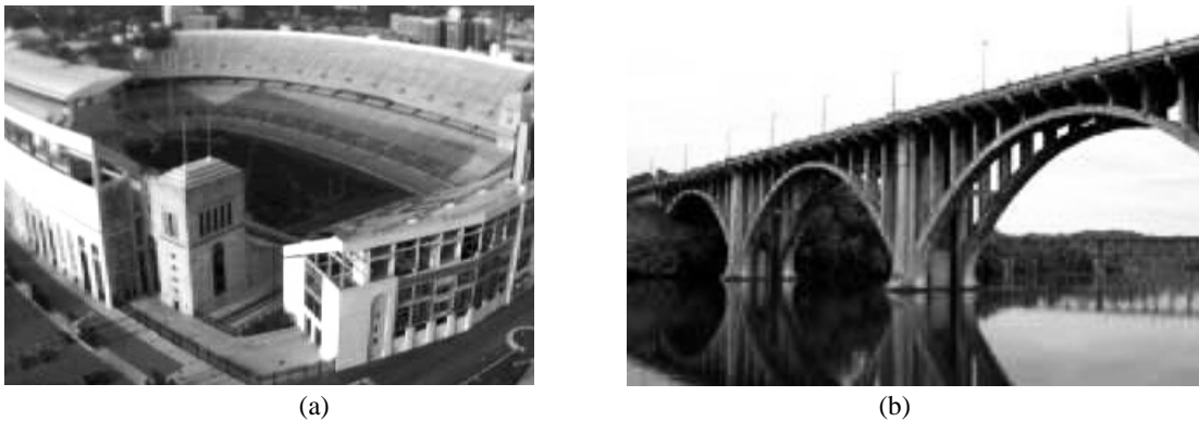
Figura 2.16: Ohio State University Stadium (2005) (a) y Henley Street Bridge (2004) (b).
