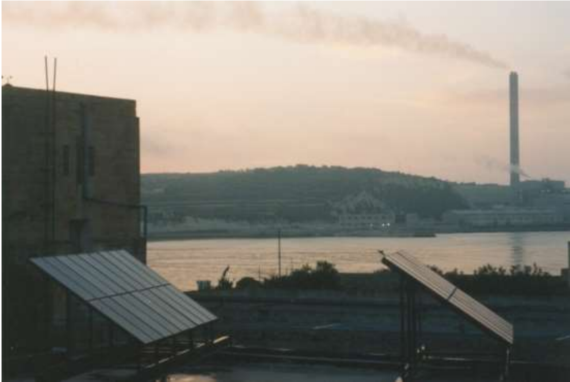
Figure 1: A 1.8 kWp grid-connected system on the roof of the Institute for Energy Technology. Delimara Power Station is seen in the background.
