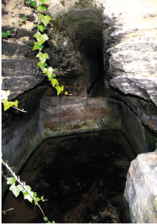
Pl. 1 A perched aquifer gallery in the San Gakbu area at Wied ir-Rum.
