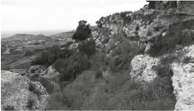
Pl. 13 The badly weathered footpath giving access to the presumed San Ġakbu cave church.
