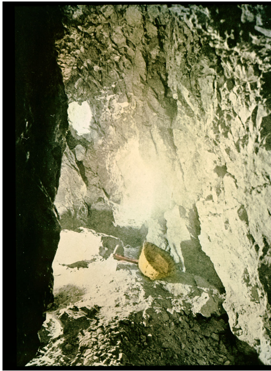
Fig. 7. The front (and main) area of Cave 1Q with original entry to the left and new/expanded entry to the right. Note the basket which shows scale, the narrowness of the cave and unevenness of the cave walls and debris on the ground. Courtesy of Oberlin College Library Special Collections, tinted image from DJD I, Pl. I:2. Reproduced courtesy of Oxford University Press and Oberlin College.
