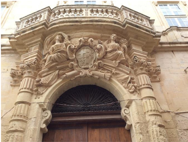
Figure 16. The easily carved Lower Globigerina Limestone effortlessly lent itself to elaborate and profuse Baroque sculpture. An extravagant doorway in the old city of Rabat (Malta).
