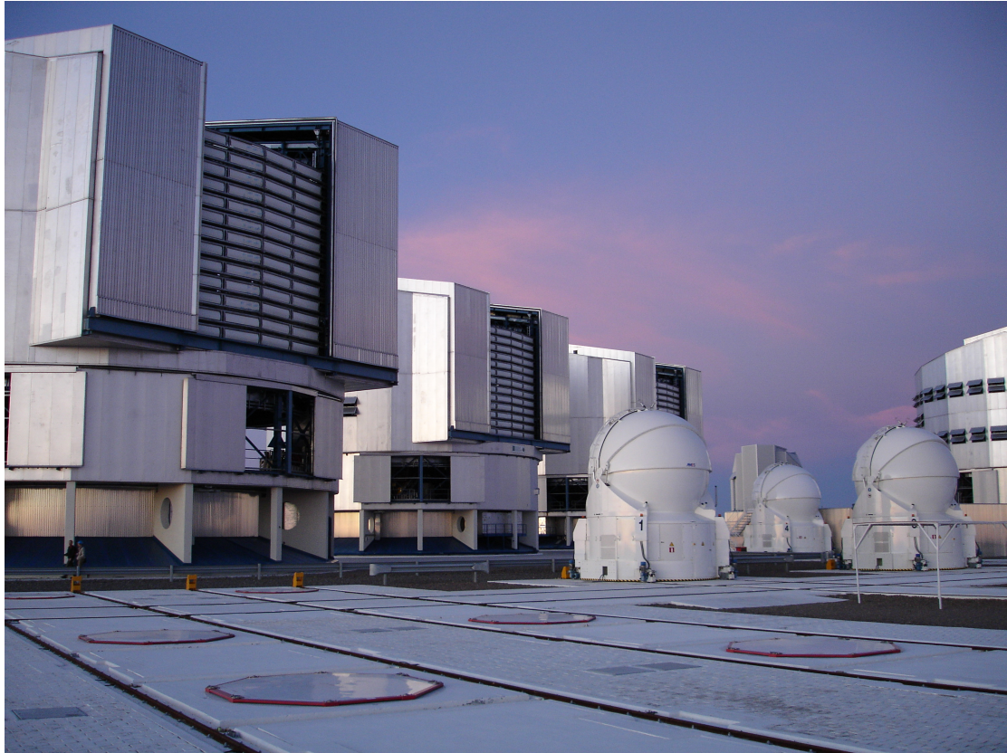
Figure 1: The Very Large Telescope observatory features four 8.2 metre unit telescopes, four 1.8 metre auxiliary telescopes, and the infrastructure for performing optical interferometry. Image Credit: S. Kraus
