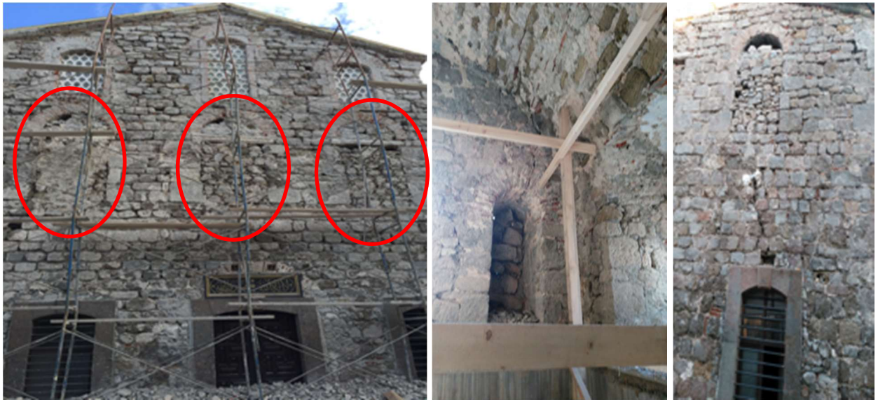
Fig. 5. Views of closed window openings on the exterior walls
