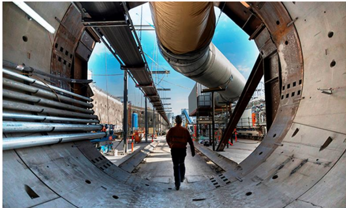
a. Realistic view of a rail tunnel
