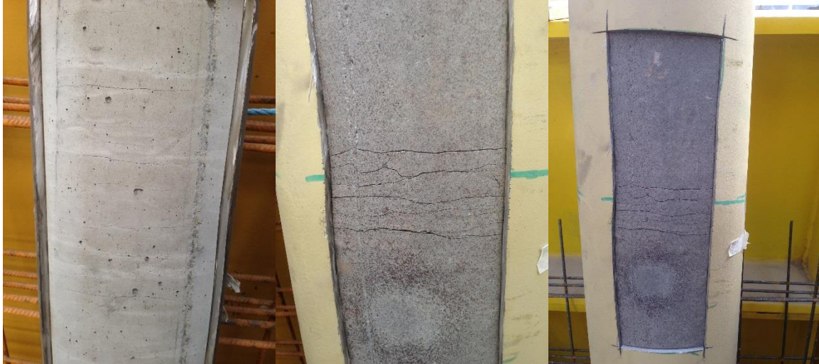
Figure 6. Tensile cracks after removing of steel tube steel
