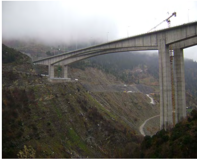
Figure 4.3: The ravine bridge of Metsovo
