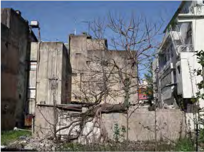
Plant at 84th Street, Jeonju, 2012.
