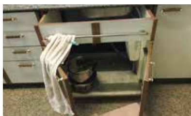
Fig. 4 A cupboards that can be taken out and move to higher place (No.11).
