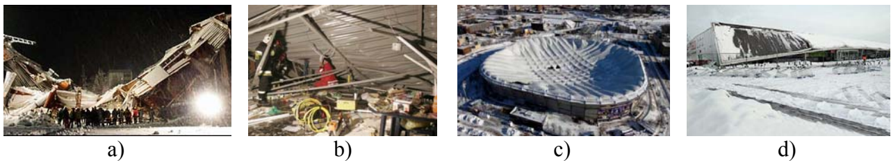
Fig. 1. Recent structural collapses due to snow accumulation (Sources: Reuters, CSBnews, CNN, dailymail.co.uk)
