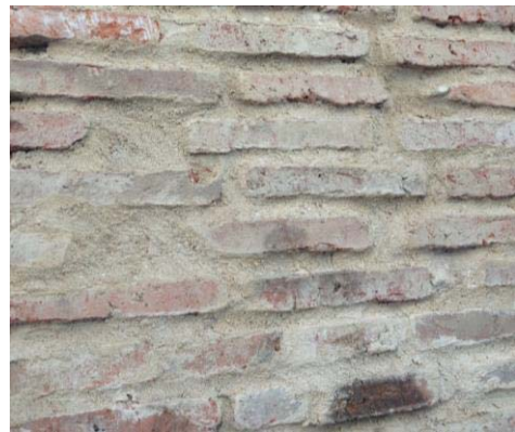
Figure 4. Detail of a brick vaulted ceiling.
