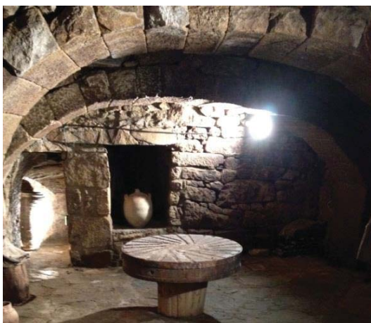
Figure 5. Segmental arch.
