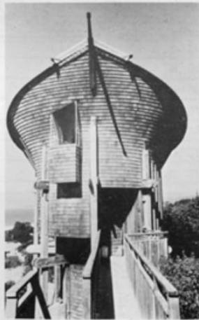
10 The architect Val Agnoli, whose father was a carpenter, built this California house by himself in eighteen months. (Photo : S. Goutman and J. Guynet, Paris).
