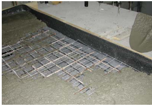
Figure 2 - Final concrete layer of the floating floor.
