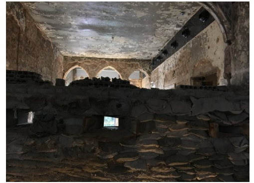
Fig. 28b: Barakat building: Trincee
