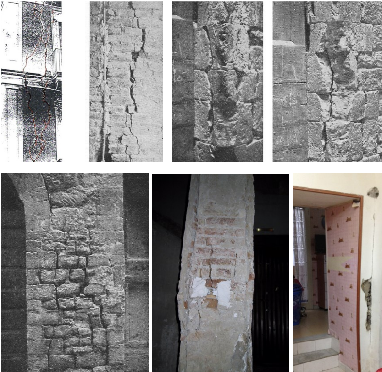
Fig. 1.5 - Some typical failure modes of the third type: crushing of the material occurring when the compressive stress is close to the compressive strength of the material.
