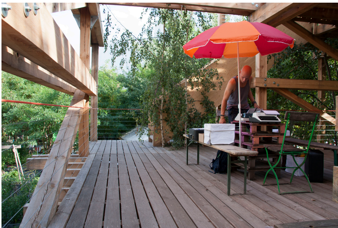
Fig.37. First floor open-air room in Die Laube. Users can add functional elements in order to customize its spaces, Berlin, Germany (author's archive, 2016).
