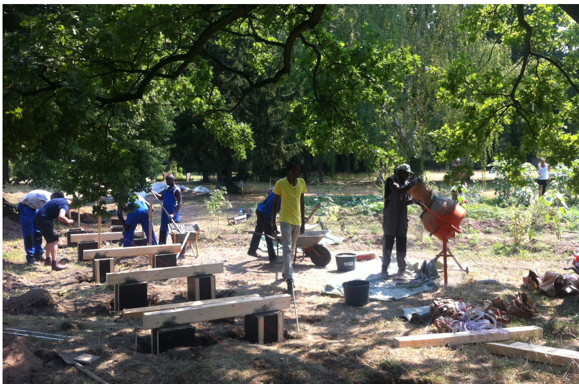
Fig. 21. The construction of the footbridge-promenade, Berlin, Germany (Die Gärtnerei Archive, 2016).
