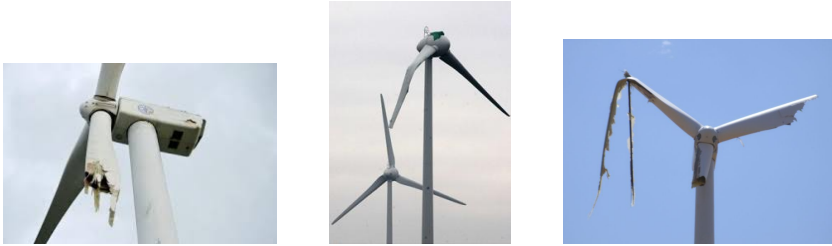
Figure 4.1: Damage effects on operating wind turbines
