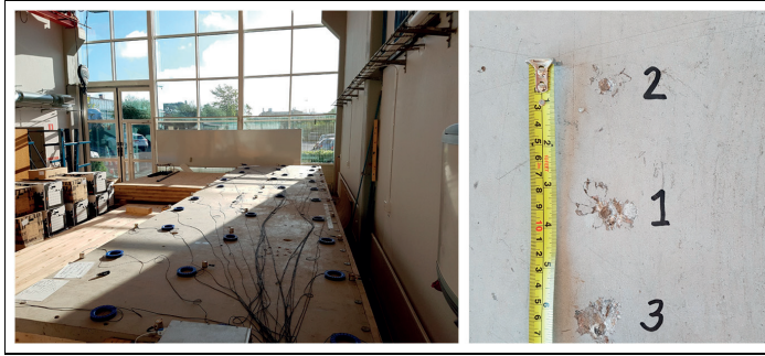
Figure 2. (Left) Photograph of the floor slab and the laboratory hall. Not all transducers seen in the photograph were used in this study. (Right) Close-up of the damage to the concrete. A ruler is included for reference.
