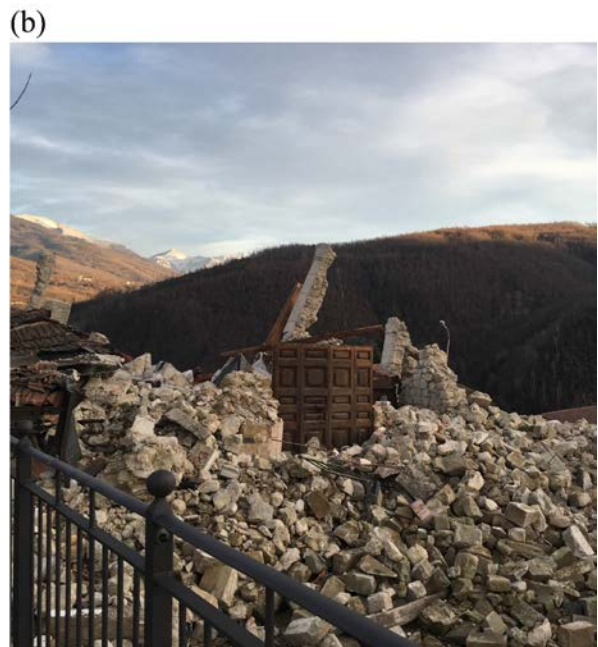
Figure 9. The local church: (a) after the first earthquake; and (b) after the entire sequence.
