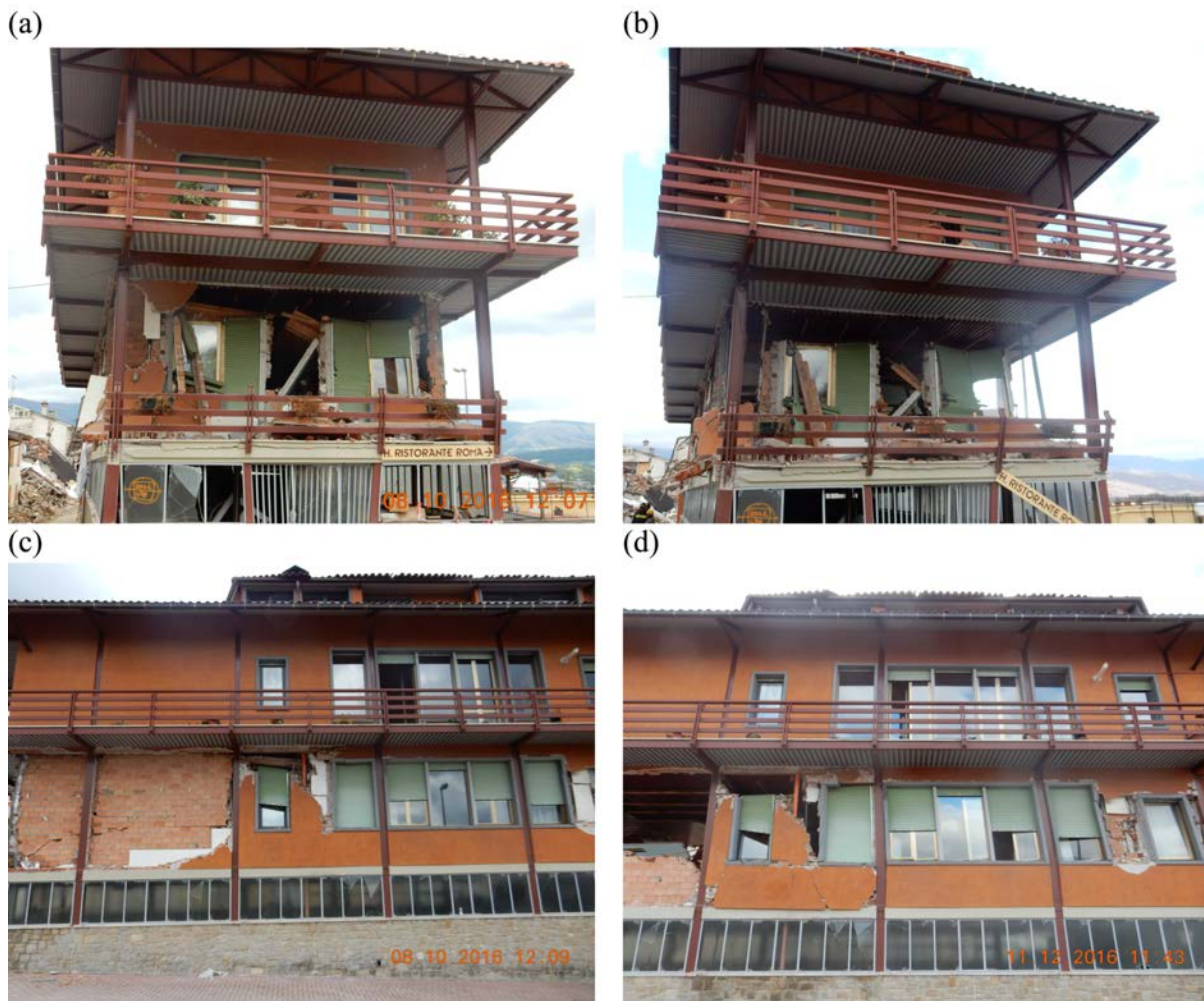
456 Figure 16. Steel residential building. (a,c) Limited damage after the 24 August earthquake and (b,d) 457 extensive damage of the infill panels at ground level with evident residual drift after the entire 458 sequence.
