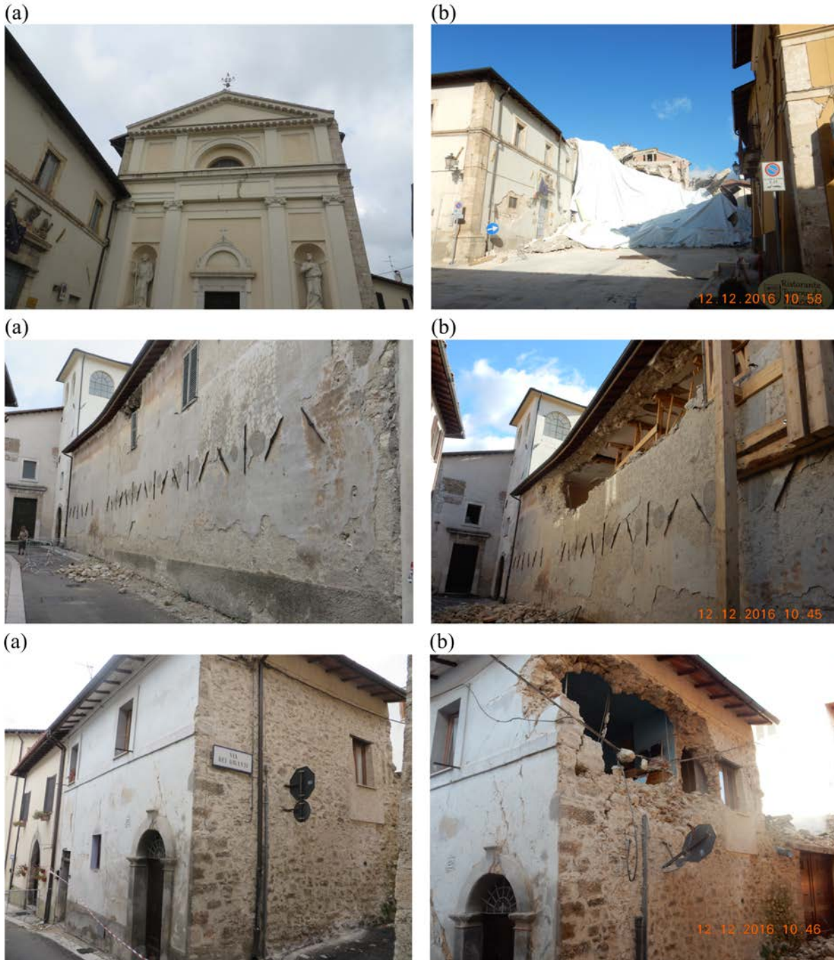
551 Figure 20. Seismic damage observed in characteristic masonry buildings (a) after the 24 August 552 earthquake and (b) at the end of the entire seismic sequence.
