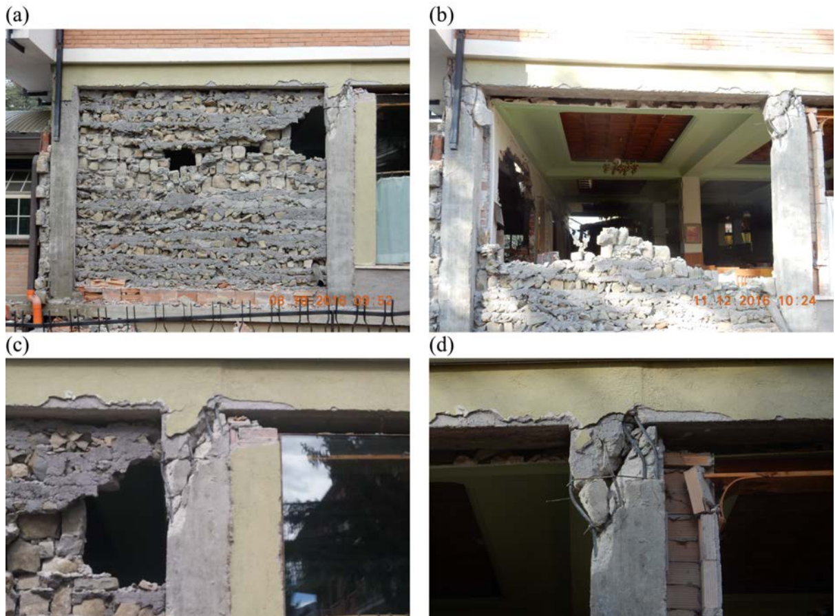
446 Figure 13. Reinforced concrete residential building (a,c) after the 24 August earthquake and (b,d) 447 after the entire sequence. (a,b) External infill failure and (c,d) shear failure at the column top.
