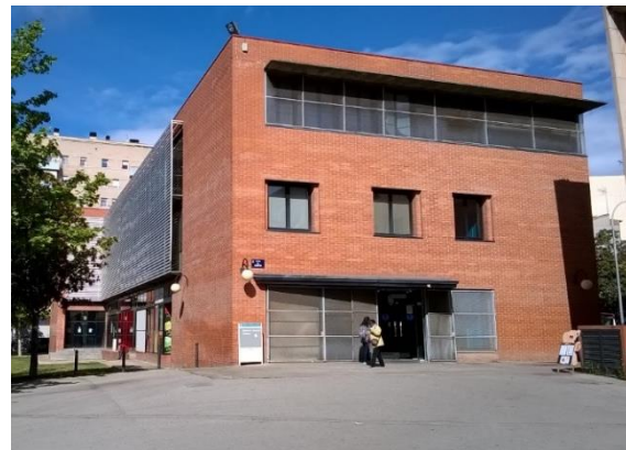
Fig. 1 – The south east façade of the UPC Terrassa library building
