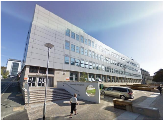
Fig. 2 – The Smeaton Building in Plymouth, UK
