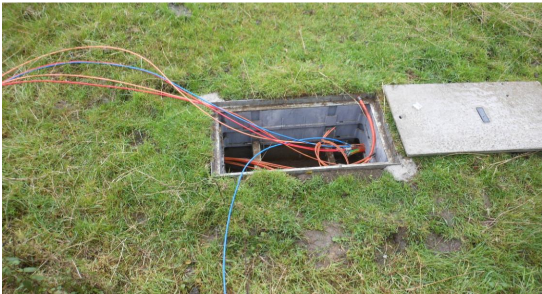
Photo 5 - 1 Partially completed fibre cabling, being installed by B4RN volunteers
