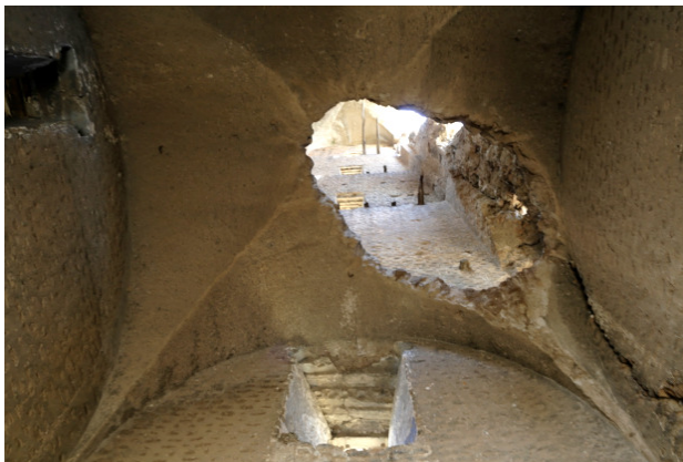
Figure 3. T. Maggiore cross vault and middle wooden ceilings
