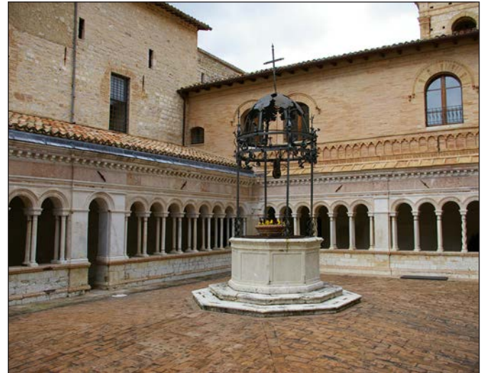
Fig. 5. The cloister of Sassovivo Abbey in 2014 after restoration and conservation campaigns. Photo by Eleonora Scopinaro
