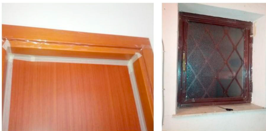
Figure 2 – Doors and windows sealing by plastic and paper scotch, simulating air-tight doors and windows.
