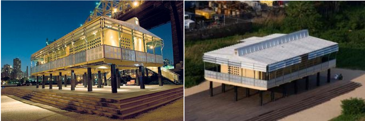
Figure 2-13: The original Prouvé house prototype erected in Congo was dismantled, returned to France and restored. Source: http://bare-minimums.blogspot.it/
