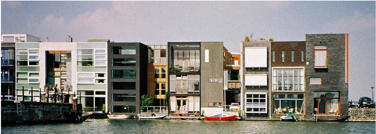
Figure 2-7: The Scheepstimmermanstraat project in Amsterdam is an example of user participation in housing. Source: Wikipedia.
