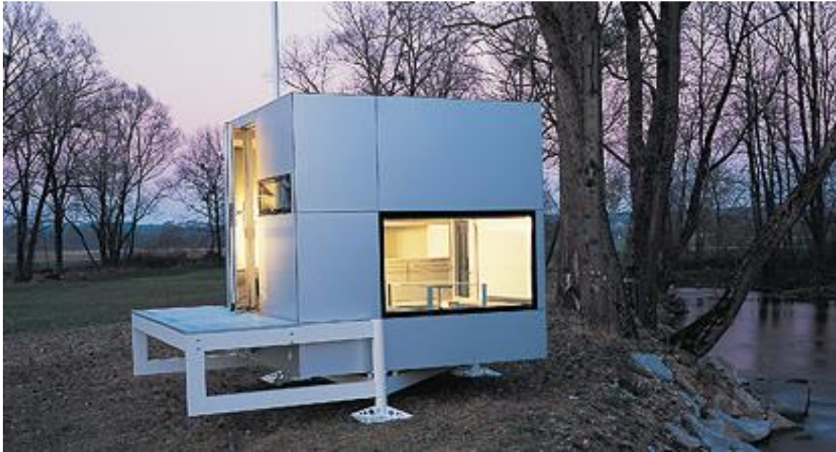
Figure 3-9: Developed for short stays, completely off-site fabrication. Source: http://www.microcompacthome.com/
