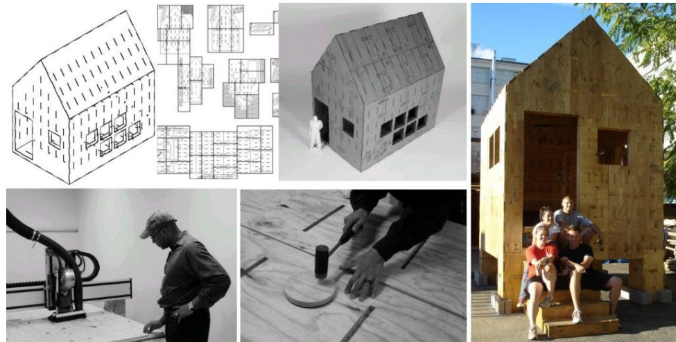
Figure 3-2: Shape grammars used to design vocabulary of Instant cabin. Source: Sass, 2005
