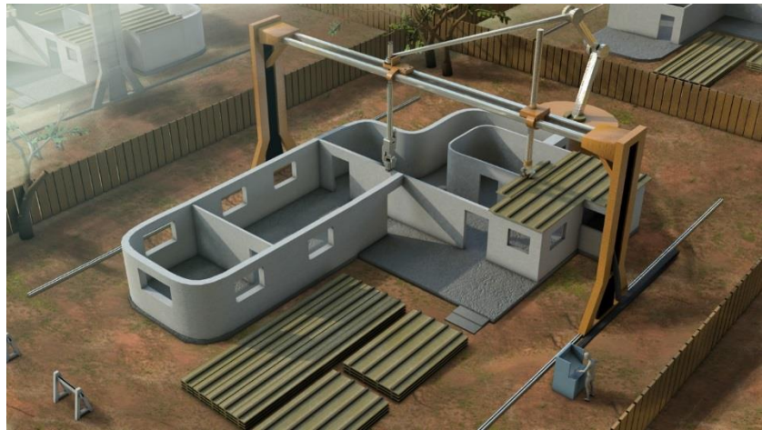
Figure 2-17: Contour Crafting, a system developed by Professor Behrokh Khoshnevis.
