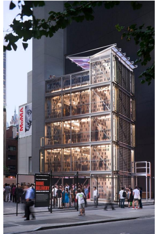
Figure 3-11: Multistory prototype built off-site completely in BIM. (Source: KeiranTimberlake, 2015)
