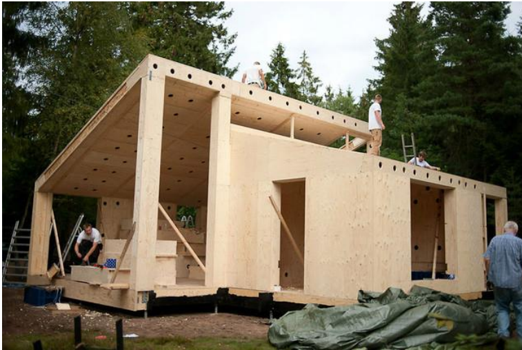
Figure 3-12: On-site digital fabrication using a mobile production facility. Source: Facit Homes
