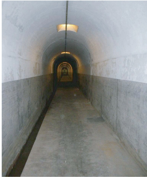
Figure 4. A picture of the concrete tunnel where propagation measurements were taken.
