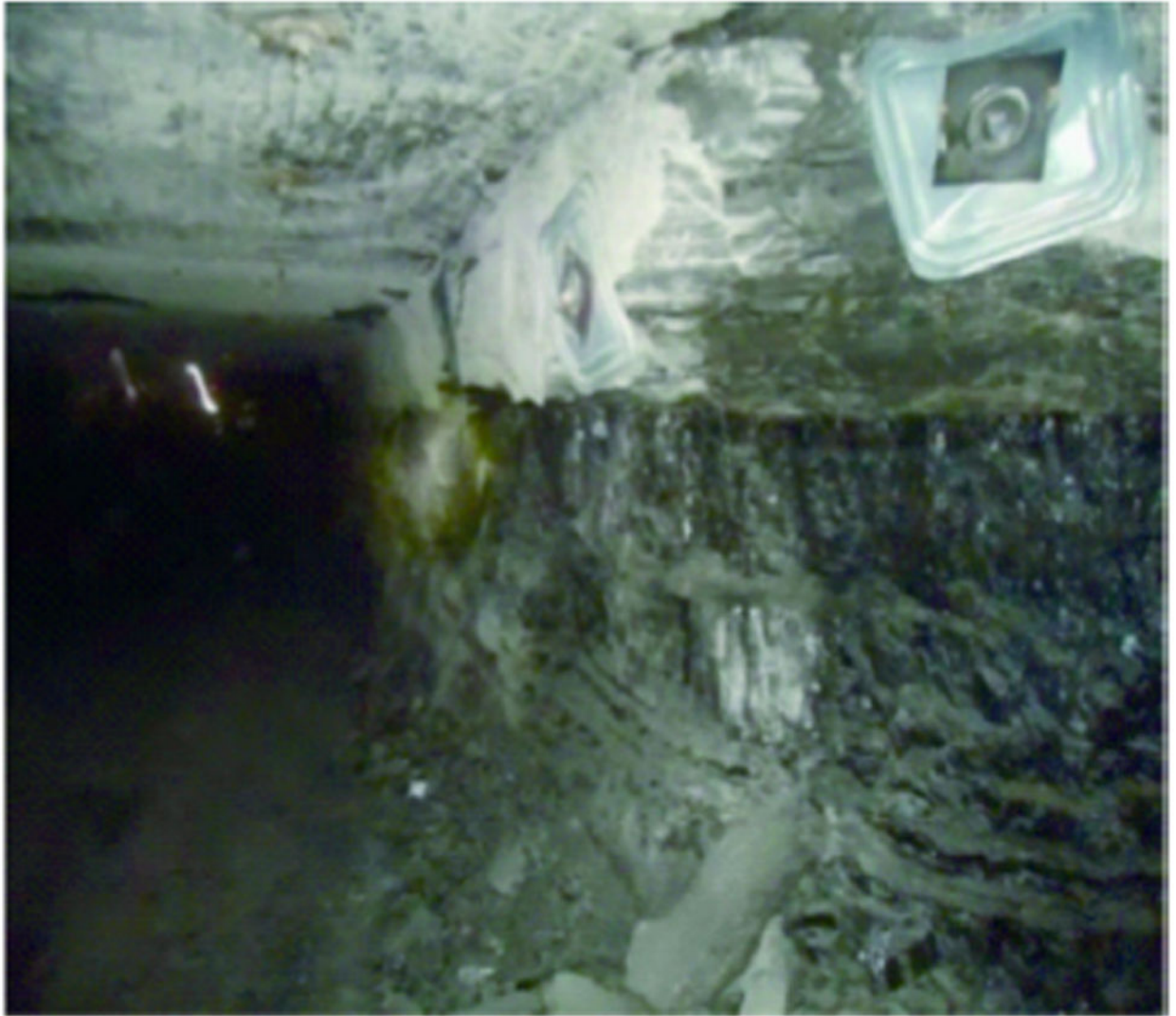
Fig. 17. Conditions of roof and pillar in the lower seam before retreating.
