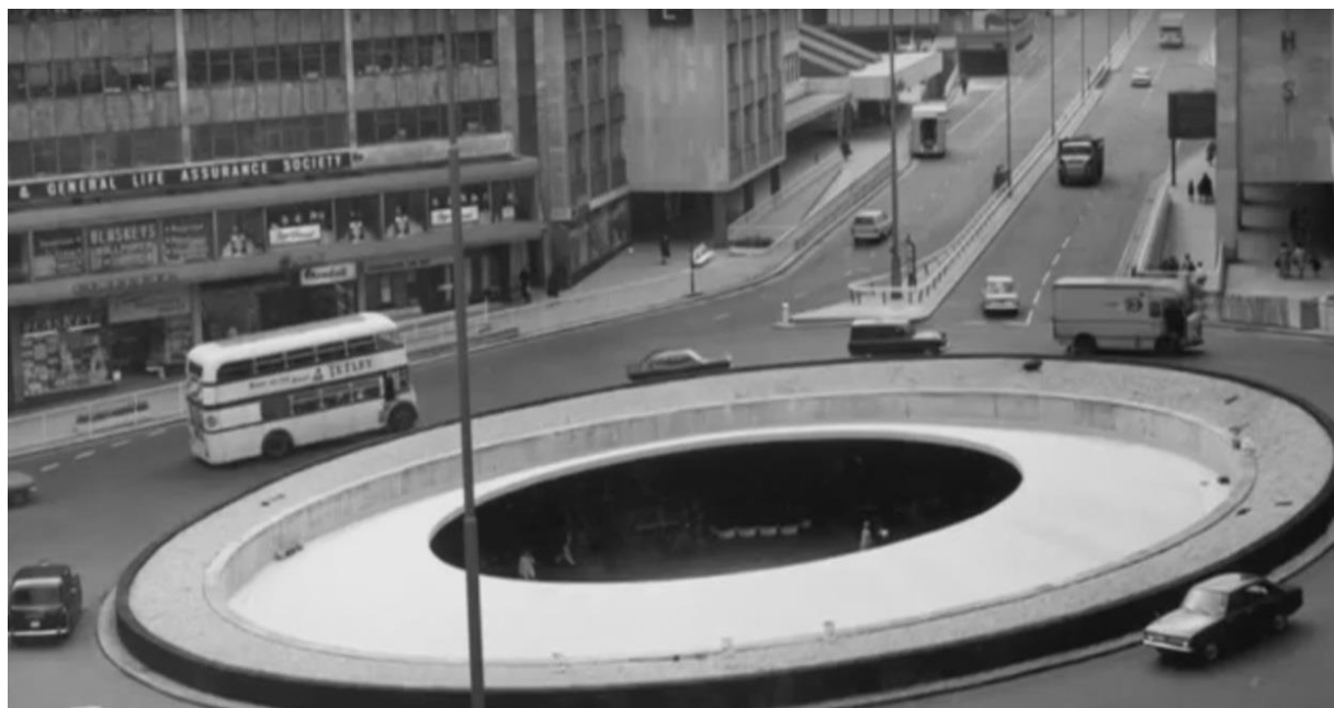
Figure 2.2: Aerial view of the Hole in the Road. Late 1960s. Exact date unknown.
