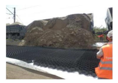
Figure 2.9 Geocell-Geotextile Hybrid System
