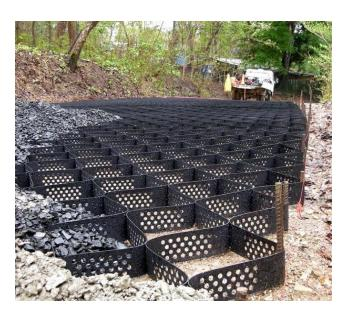
Figure 2.5 Geocell Application in Roadway
