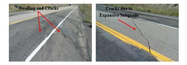
Figure 1.3 Pavement Distresses on US 95 pavement section (MP 16.7 to MP 18.5) due to expansive subgrade
