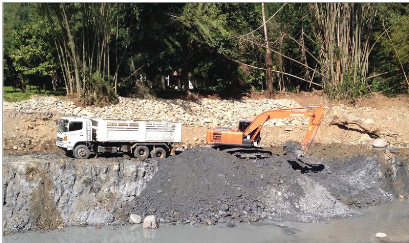
Fig. 14 Photograph during January, 2016 excavation of pit into dark-gray sheared quartzite, sheared pieces embedded in gray gummy clay. Resulting reservoir is ~ 12 m deep. This clayey material apparently lies within or beneath the quartzite just east of the hot springs. No bedding planes observed (clean exposure is left side of photo). No pyrite or visible mineralization observed in the clay or rock. Location is 0516550E, 2207200N
