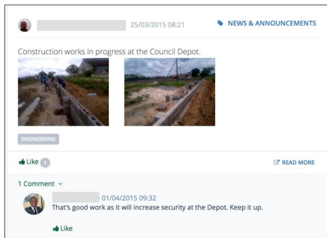
Figure 3 A member from the council posting about progress on a construction project
