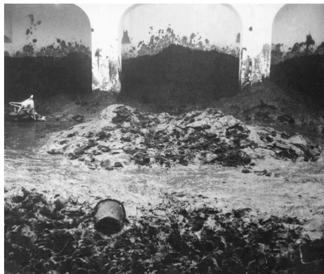
Figure 3. House in mud. Mud installed in a gallery (Sierra, 2005, p. 494)
